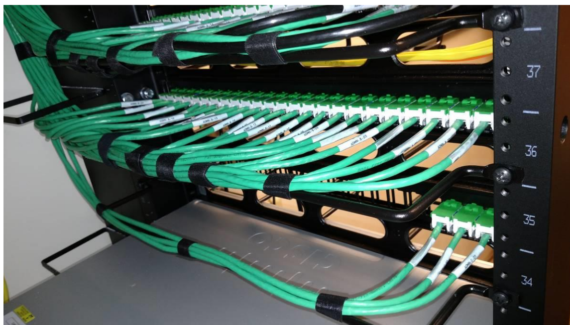
Detail 01. Proper routing and support of cables on rear organizer. Where possible route 12 cables from right side and 12 cables from left side. This rack in picture did not have right side organizer.
